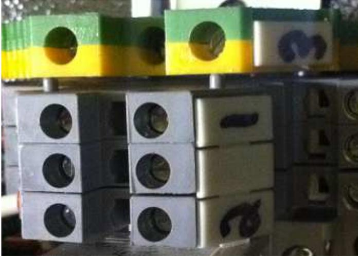
4. It is important to use a strain relief on the incoming cable to avoid strain on the terminal strip connections.
